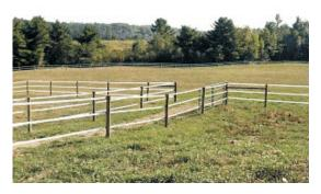
FAST FENCE™ Horse Tape™ electric fences are also used for subdivision and cross fencing. From two up to five strands may be used with figerglass Superrod™ Posts depending on conditions and personal preference.
